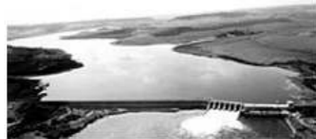
Igarapava Hydroelectric Power Plant: Nominal head: 17 m Plant Installed power: 210 MW Number of Turbines: 5 double regulation bulb turbines Nominal unit generation power: 43.6MW Rotation speed : 112,5 rpm Runner Diameter: 6,0m
